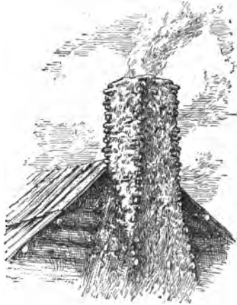
A cat-and-clay chimney, made of small split sticks embedded in layers of clay mortar.
